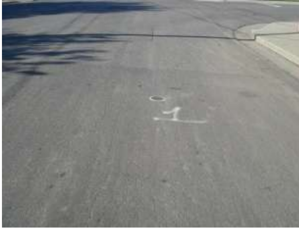
a. Pavement condition around core #1
