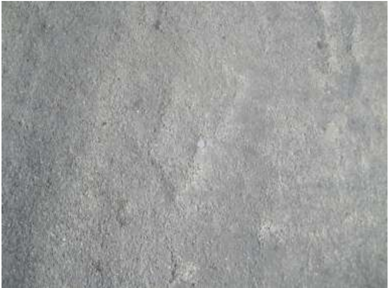
Figure 14. Crack didn't reflect through the cape seal
