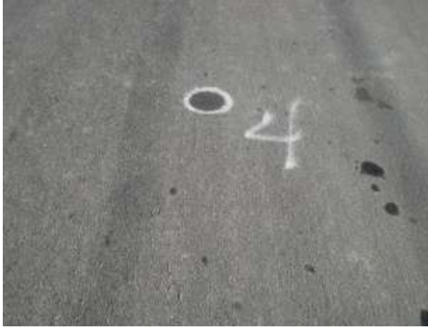
a. pavement condition around core #4
